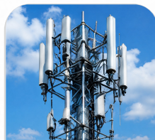
Communications System Testing
